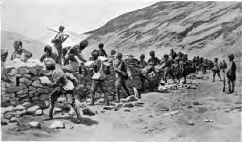
DISMANTLING LOOP-HOLED WALL AT KANGMAR.
